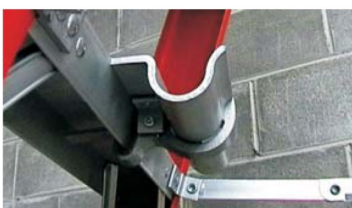
Rung Lock Assembly
